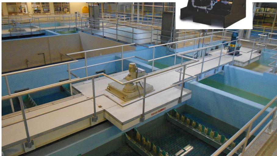
Improved polymer activation and feed at Mankato's Water Treatment Plant, through the addition of a ProMix-S polymer blending and delivery system (*inset photo*), has brought improved solids settling in the plant's softening reactor, especially at higher flows.
